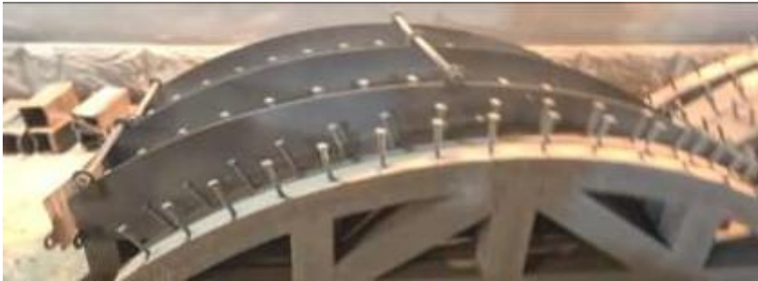
Figure 6.2: shear connector distribution
